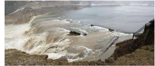
Fujinuma dam failure ( H=18.5\text{m} L=133.2\text{m} , top fill composed of poorly compacted weak sandy soils, i.e. prone to strength degradation & liquefaction)
