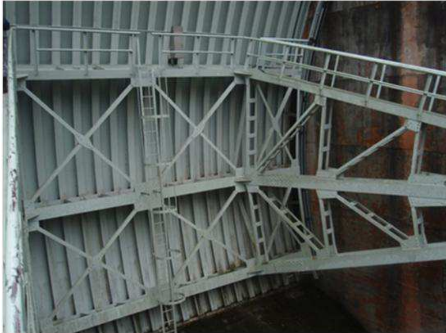
Japanese Vertically Stiffened gate; Ohtori Dam : gravity arch; Owner : J-Power; ©J-Power
